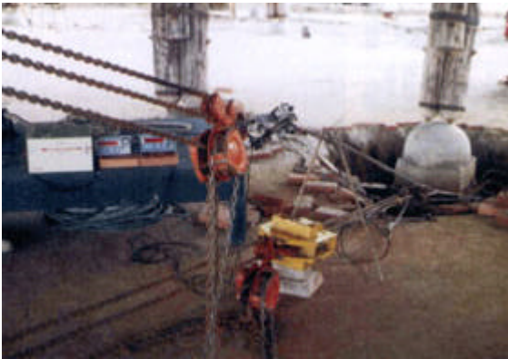
test of the foundations with chain draws
