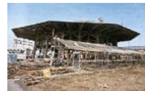
ZERI pavilion during the building
