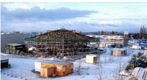
pavilion during building
