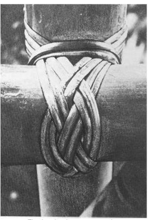
**Plait strips:** Usual plait materials are rind strips of bamboo, rattan or lianas. Soaked before use they are more pliable. When drying, the fibres shrink and the connection tightens.
