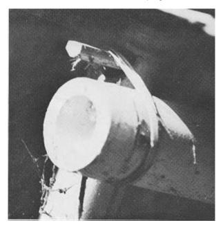
**Rope connection fixed with bolt.** The bolt keeps the conncetion in place even if the rope or cord lenghtens .
